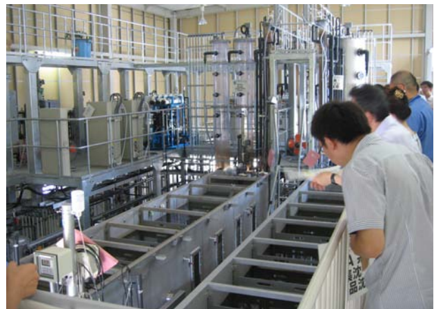
Visit to Kunijima water treatment plant
