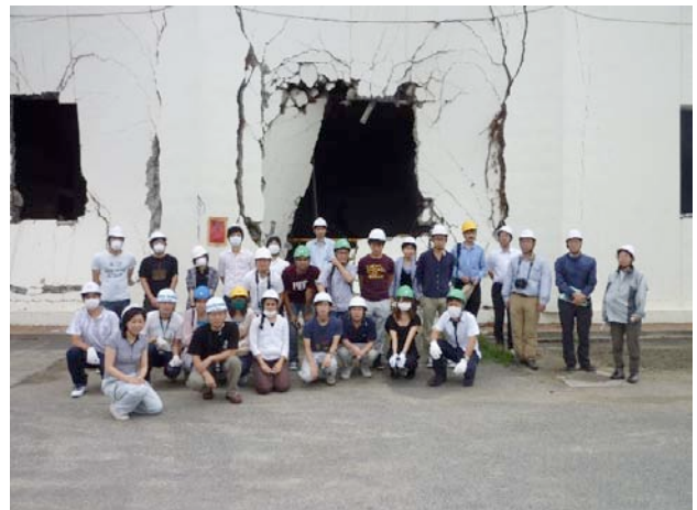
Participants of Seminar (in front of Tsunami damaged building at Minami-Gamou sewage disposal plant)
