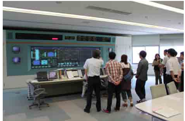
Tour of the treatment facility (Monitoring Room)
