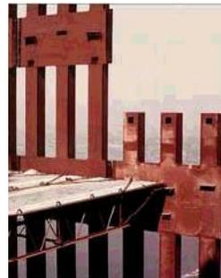
900mm deep 'open-web joists' (trusses) topped with 100mm concrete deck
